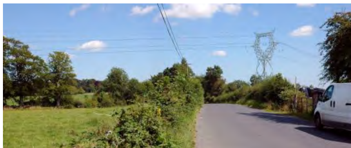
Photomontage 62 from an open section of the L4008 east of Dunderry, at a distance of 179m. This represents a worst case impact where a tower is located immediately adjacent to a road.
