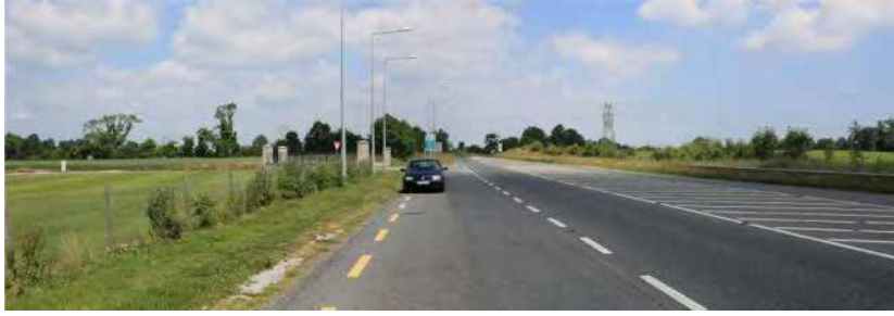
Photomontage 63 from an open section of the R161, at a distance of 407m. This represents an open view where three towers are partially visible against the skyline in a flat river valley landscape in the context of a regional road.
