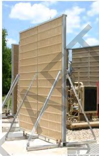
Figure 9.4: Example of a Section of Temporary Noise Barrier
